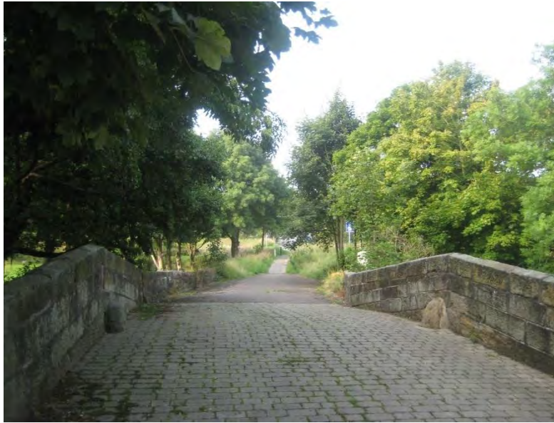
The Old Oxspring Road Bridge
