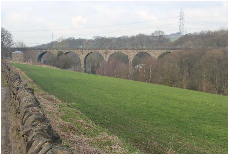
View of Viaduct, Sheffield Road opposite Eddyfield
